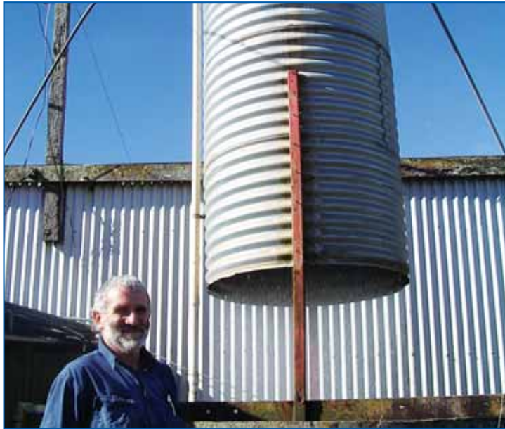
Duncan Sadler with cooling tower
