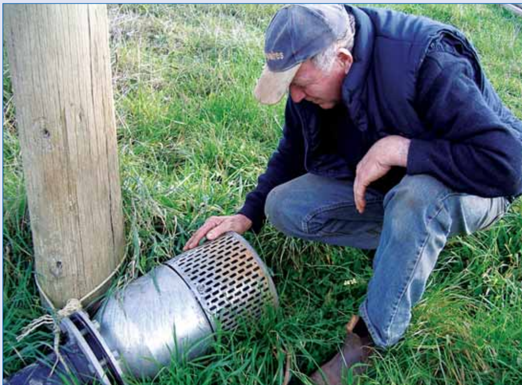
John Sadler checks a foot valve
