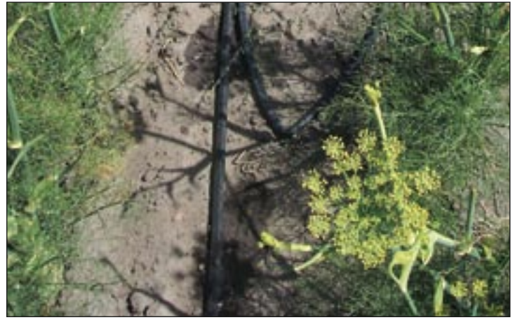
Drip irrigation system watering vegetable fennel.
