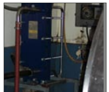
Plate cooler and vat in dairy.
